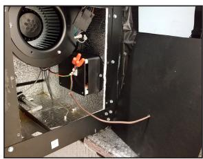
Install the evaporator access panel onto the unit using the six previously removed screws. Use cork tape or duct tape to seal around the hole which the wire was ran through.
