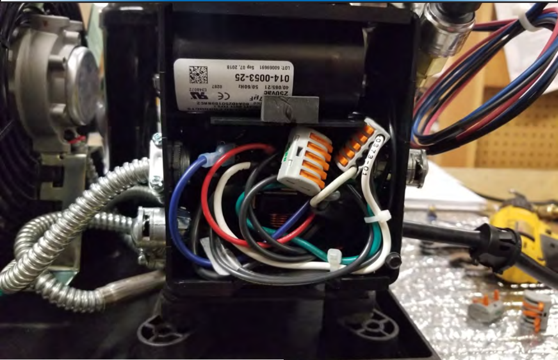
Push wires back into enclosure.
