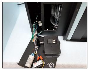
13 Cut zip ties securing wires.
